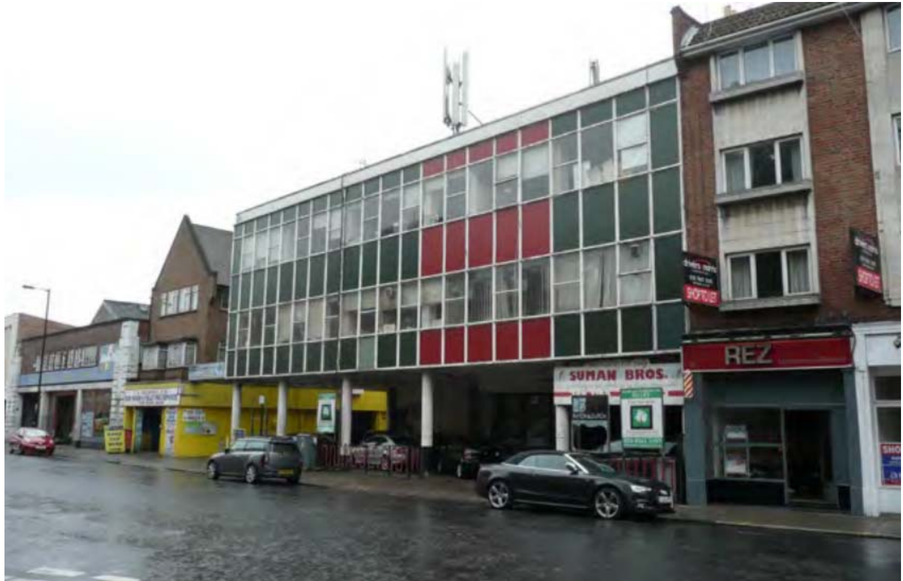
Existing front facade 2
