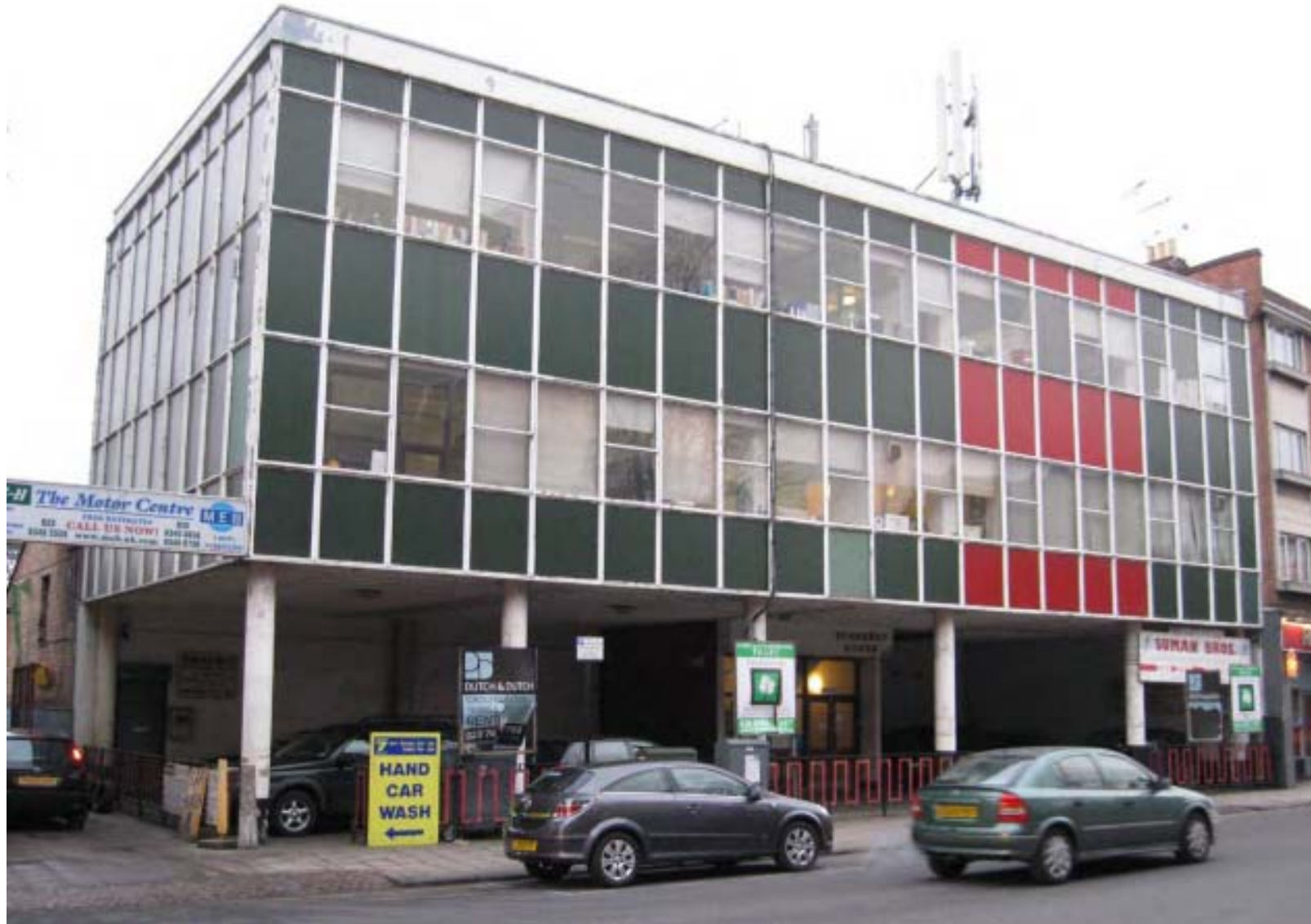
Existing front facade 1
