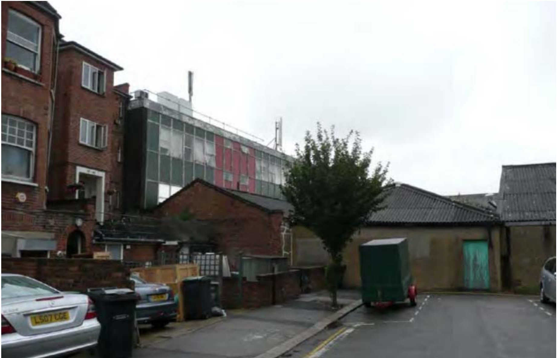
Existing rear (Fairview Gardens)
