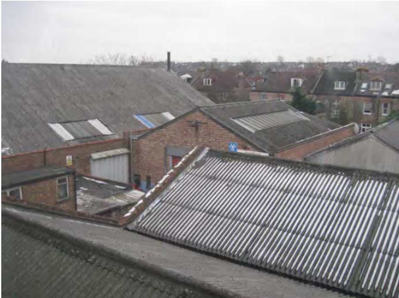
Existing warehouse roofs
